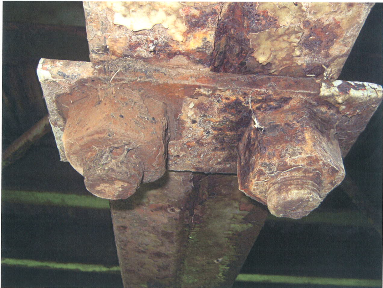
LOG C21-1.00 – L9 FLOOR BEAM HANGER PLATE
