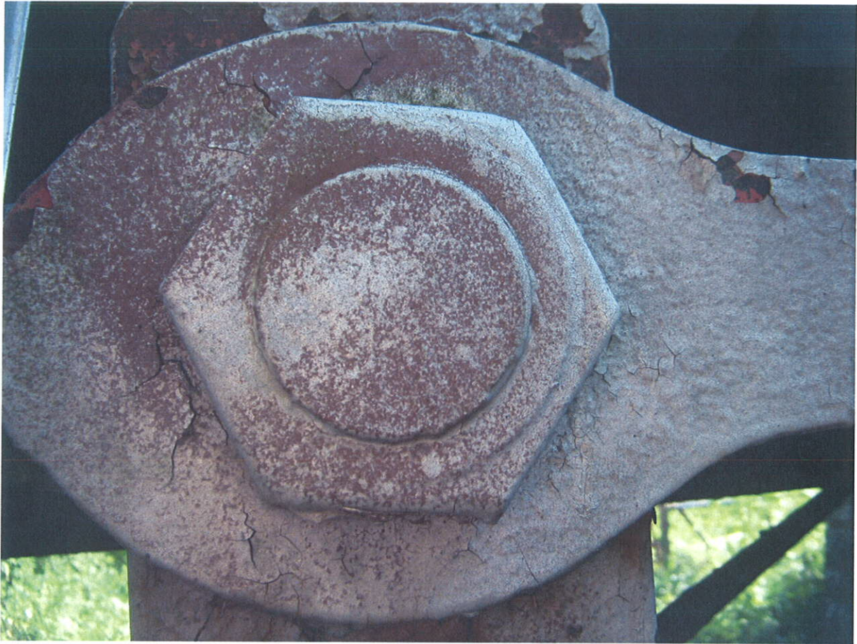
LOG C21-1.00 – L9 PIN SOUTH TRUSS (EAST END)
